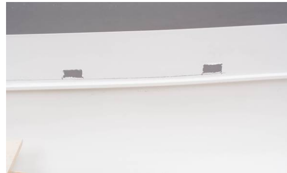
Fig. scuppers cut out, from inside
